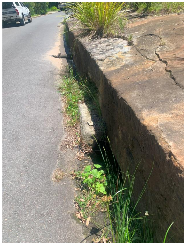
Figure 3: Water egress at the base of the rock outcrop on the northern side of The Rampart.
